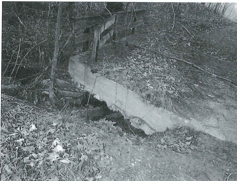
Photograph #2 - Bridge At North End Of Development
