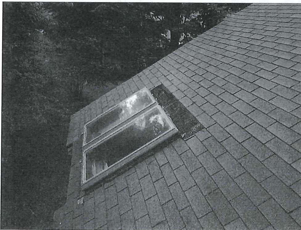
Photograph #18 - Exposed Waterproofing Membrane Above Duplex Skylight
