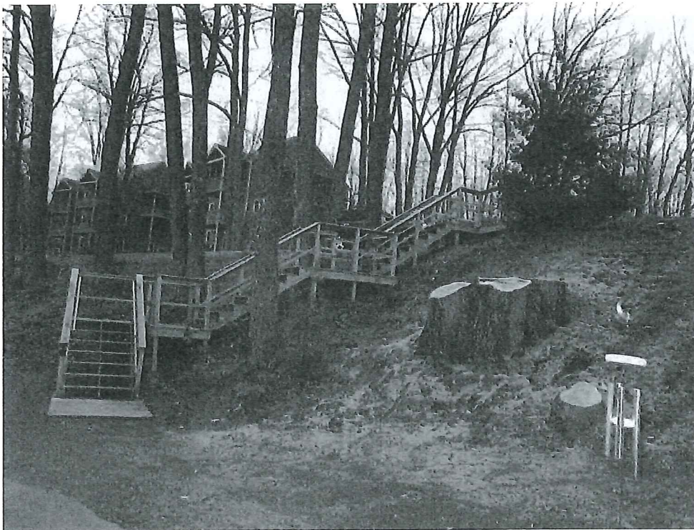
Photograph #4 - Framed Stairway
