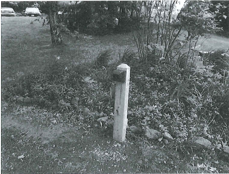
Photograph #24 - Walkway Light
