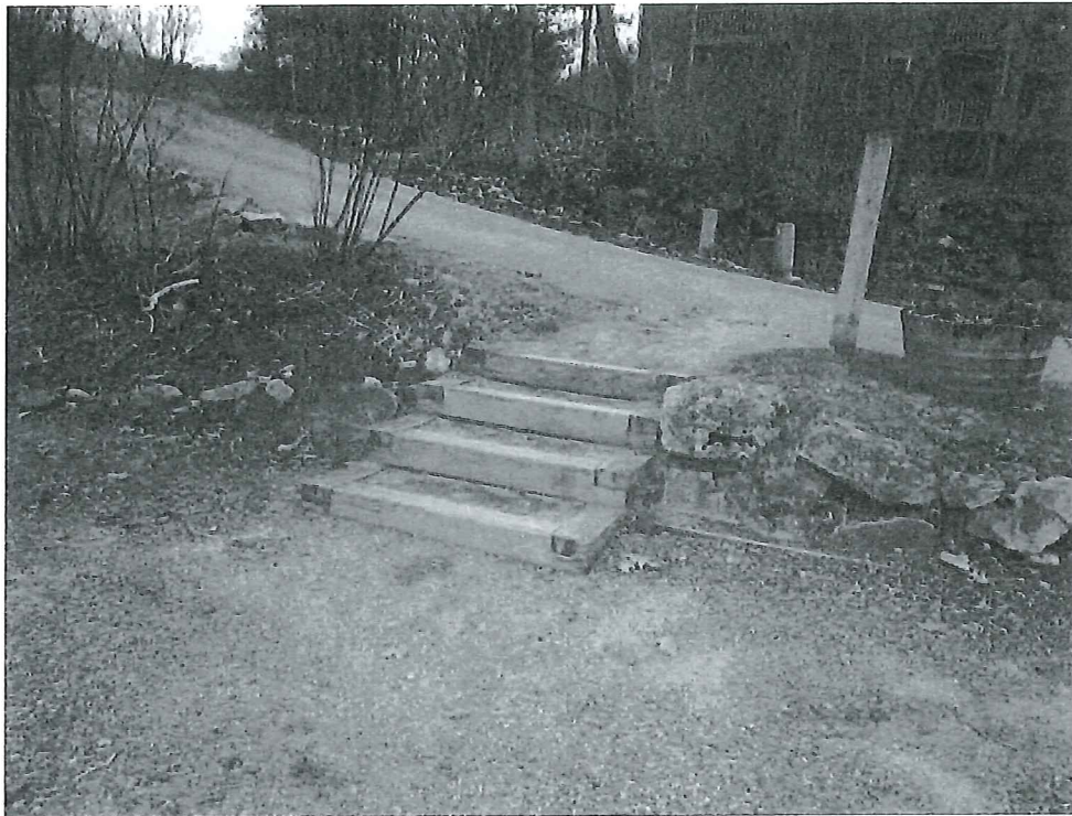
Photograph #3 - In-Fill Stairway
