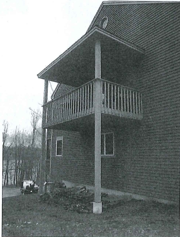
Photograph #6 - Duplex Exterior Deck
