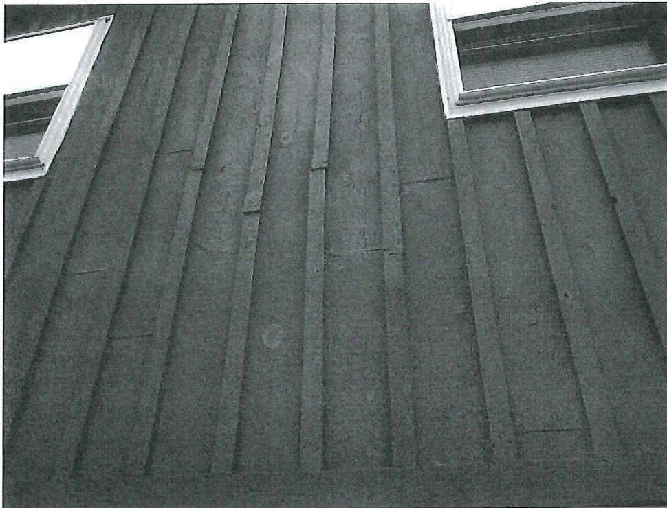
Photograph #7 - Siding On Triplex Building
